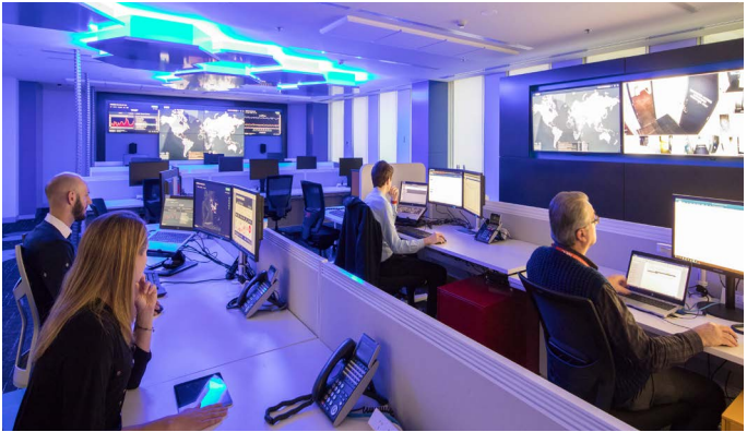
NEC's Security Operation Centre in Adelaide
